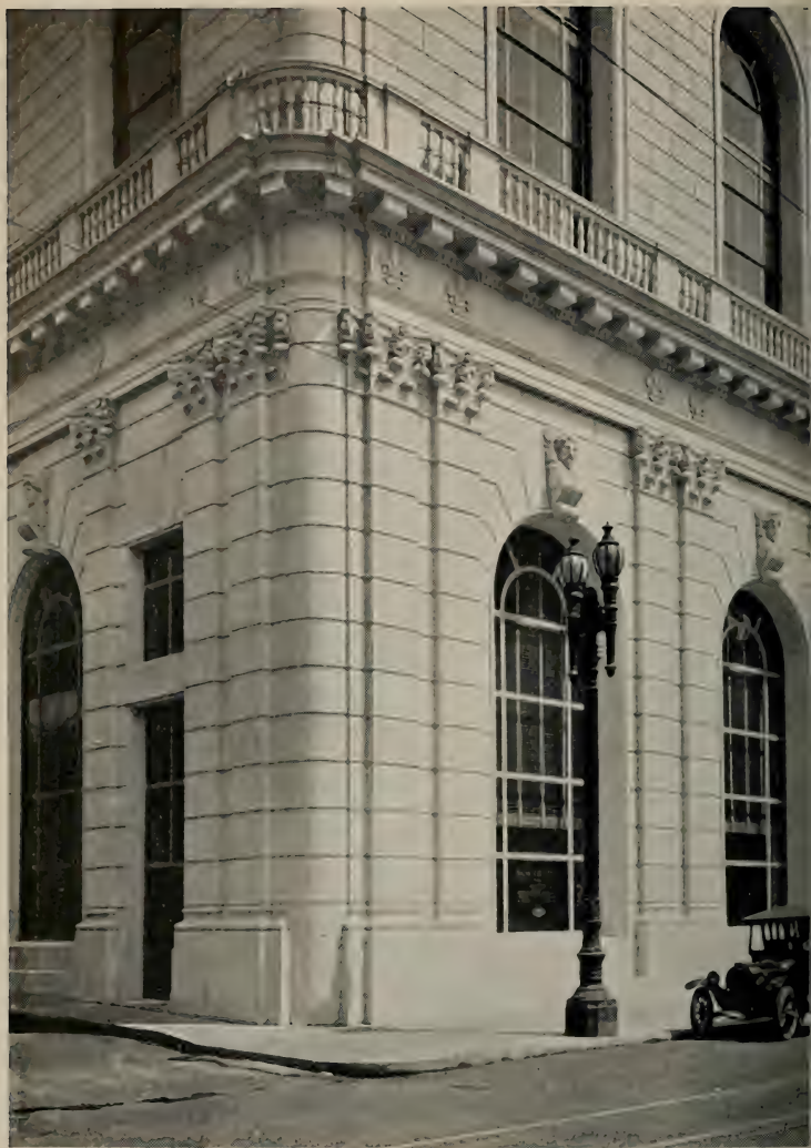
Lower Part Southwest Corner Bank of Italy Building
